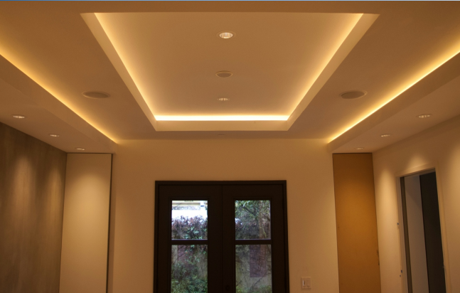
Cove Lighting using LinR12-ST-27k
